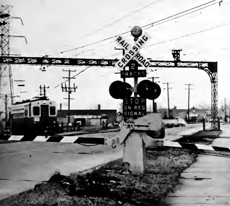
As on a main line railroad, automatic crossing gates, with interconnected motorman's signal lights, give priority to train passengers at the seven grade crossings. Rehabilitation work included installation of fifteen new gates like these at Niles Center Road.
